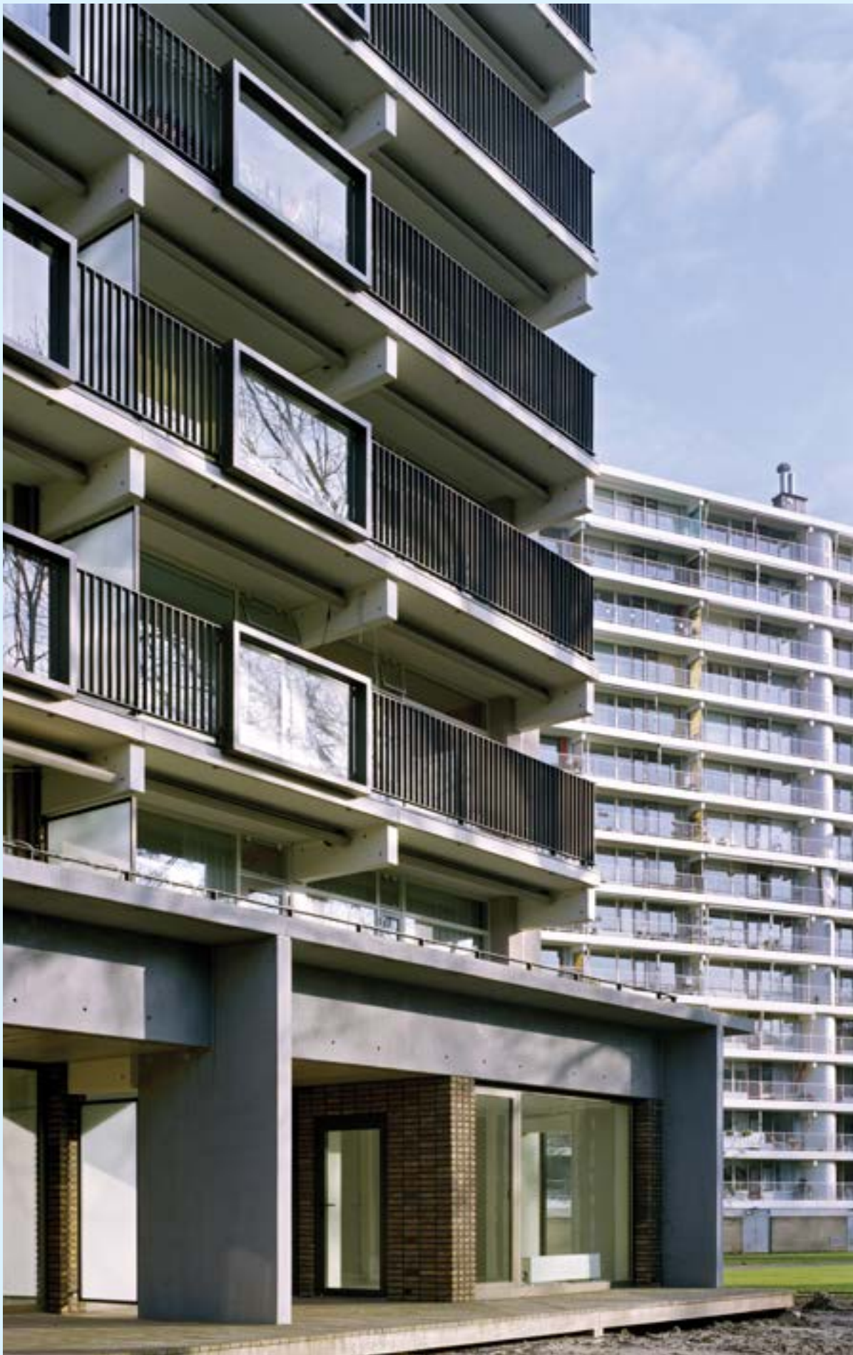
← Hans van der Heijden/Biq redesigned the Splayed Apartment Blocks in Rotterdam to better accommodate both the occupants who had lived there since the blocks were built in 1968 and those who had moved in more recently. Photograph: Stefan Müller
